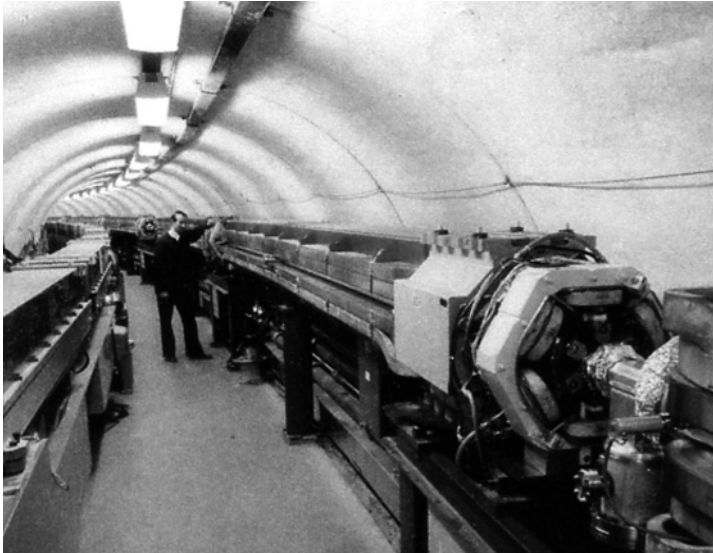
Inside the tunnel, circa 1983. (Cornell 2000)
