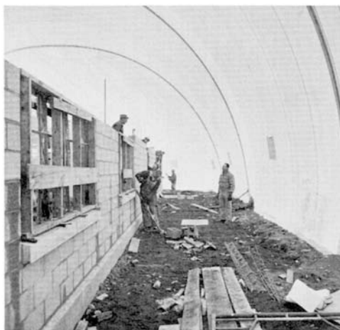
Constructing Small Building In Inflated Enclosure
