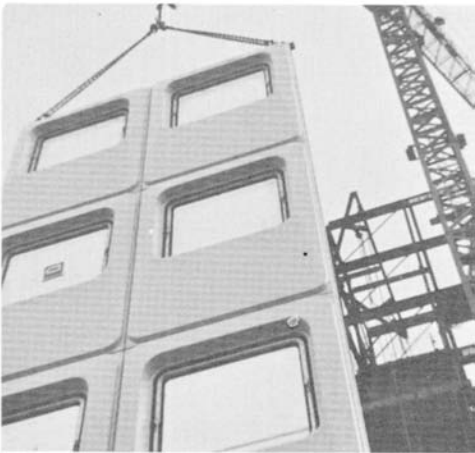
Six Preassembled Panels Erected At Once
