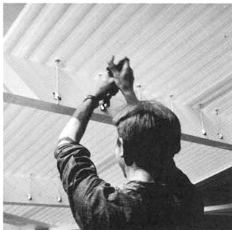
Applying Corrugated Sheet
