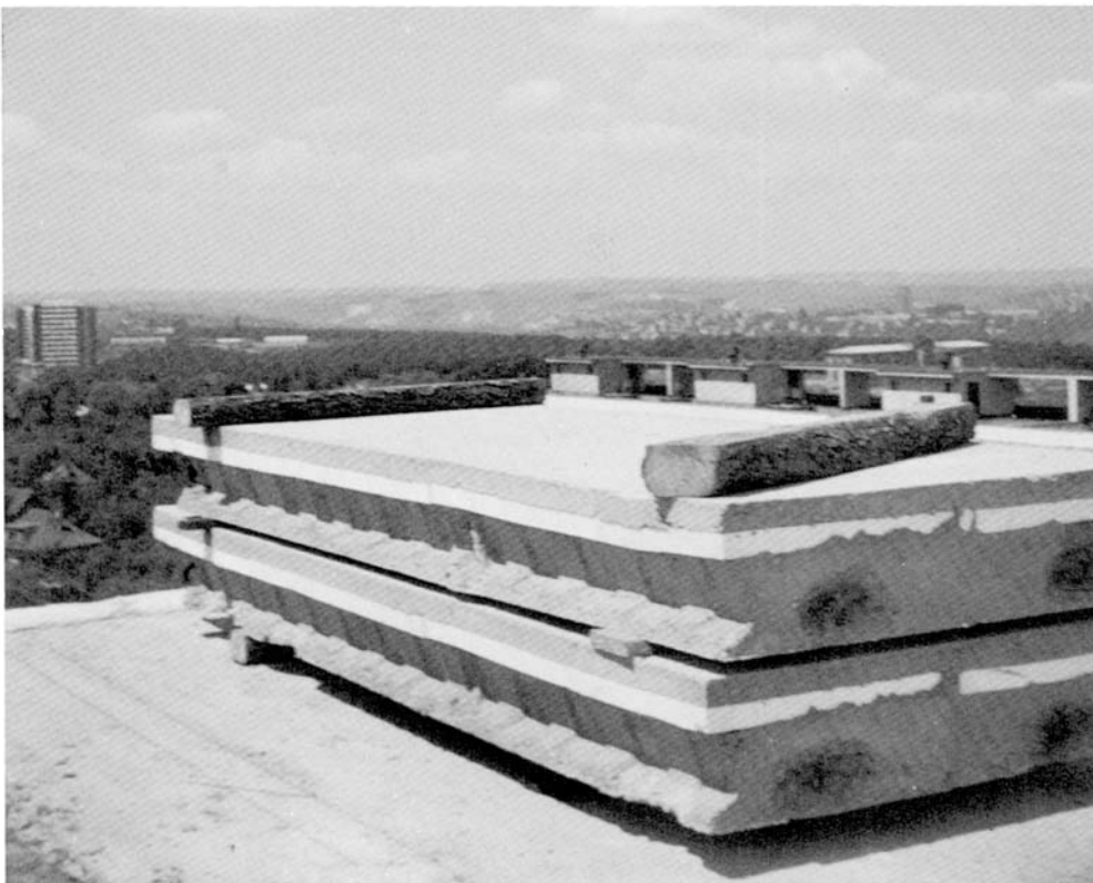
Concrete Wall Panels With Polystyrene Foam Insulating Layer, Prague
