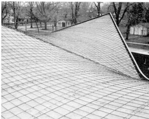
Hyperbolic Paraboloid Formed with Polystyrene Foam Planks
