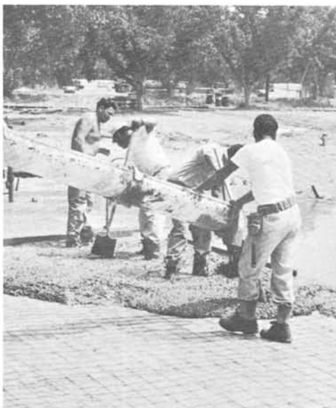
Casting Concrete on Film
