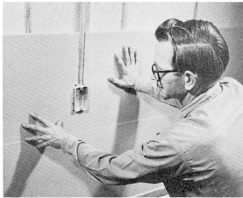
Polystyrene Foam Base for Plaster
