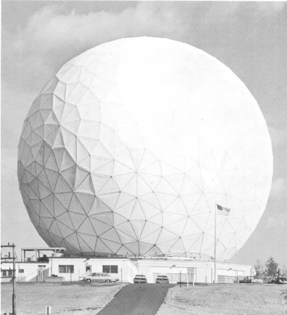
Radome, Metal Frame, Reinforced Plastic Skin
