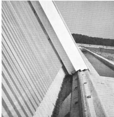
Flexible Connection, Corrugated Sheet to Support
