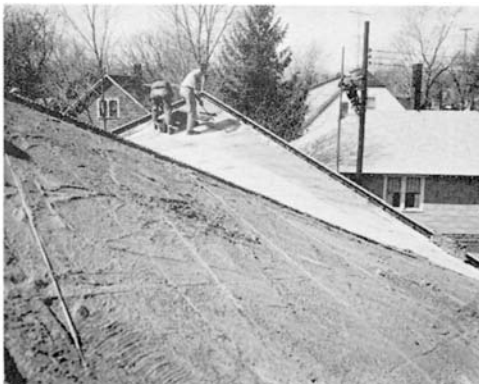
Concrete Deposited on Foam
