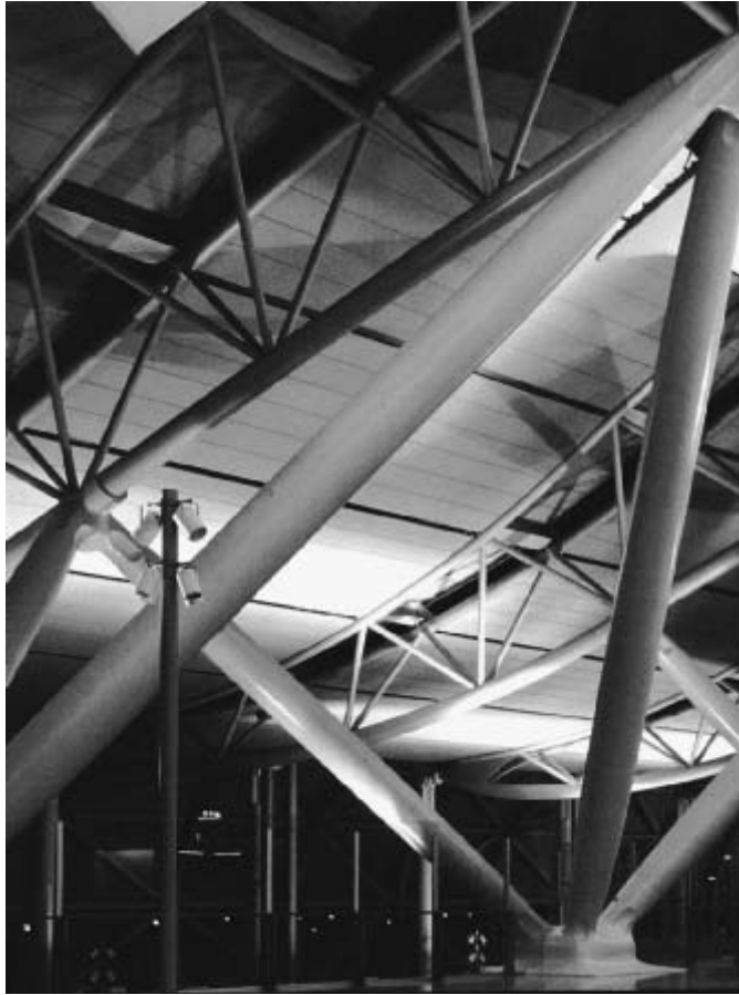
1.1. Renzo Piano, Kansai International Airport, passenger terminal.
